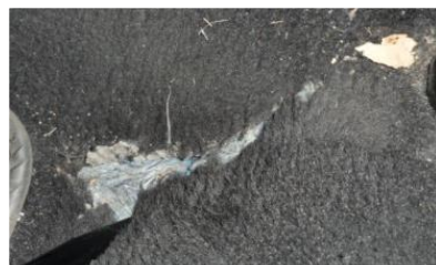
Vloerbekleding ingescheurd
